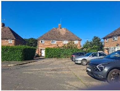
1: Looking at 9 Tenter Close from adjacent property
