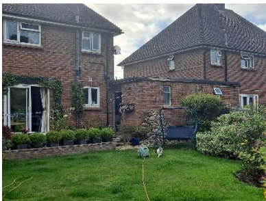
7: Rear of 9 Tenter Close showing out building that I to be retained
